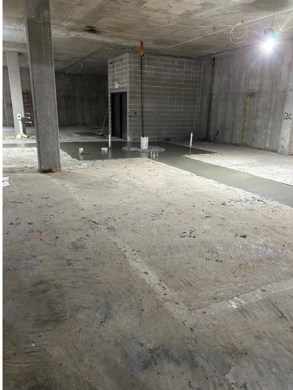
Lower Level – Plumbing Trench
