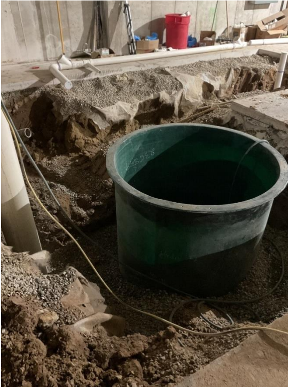
Lower Level - Sump Pit
