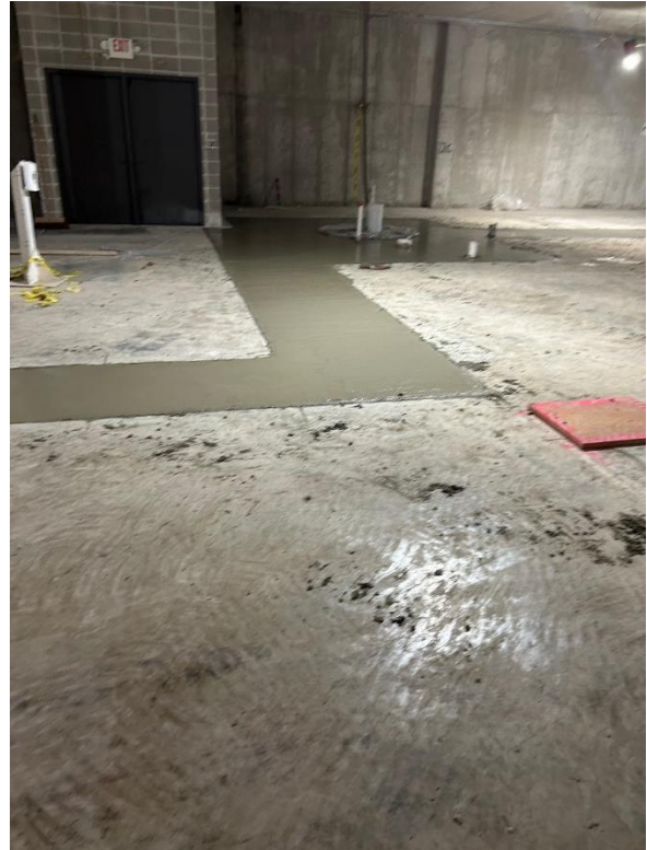
Lower Level – Plumbing Trench
