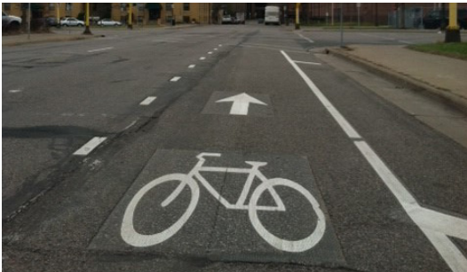
Recessed thermoplastic bike lane symbol. Alta.
