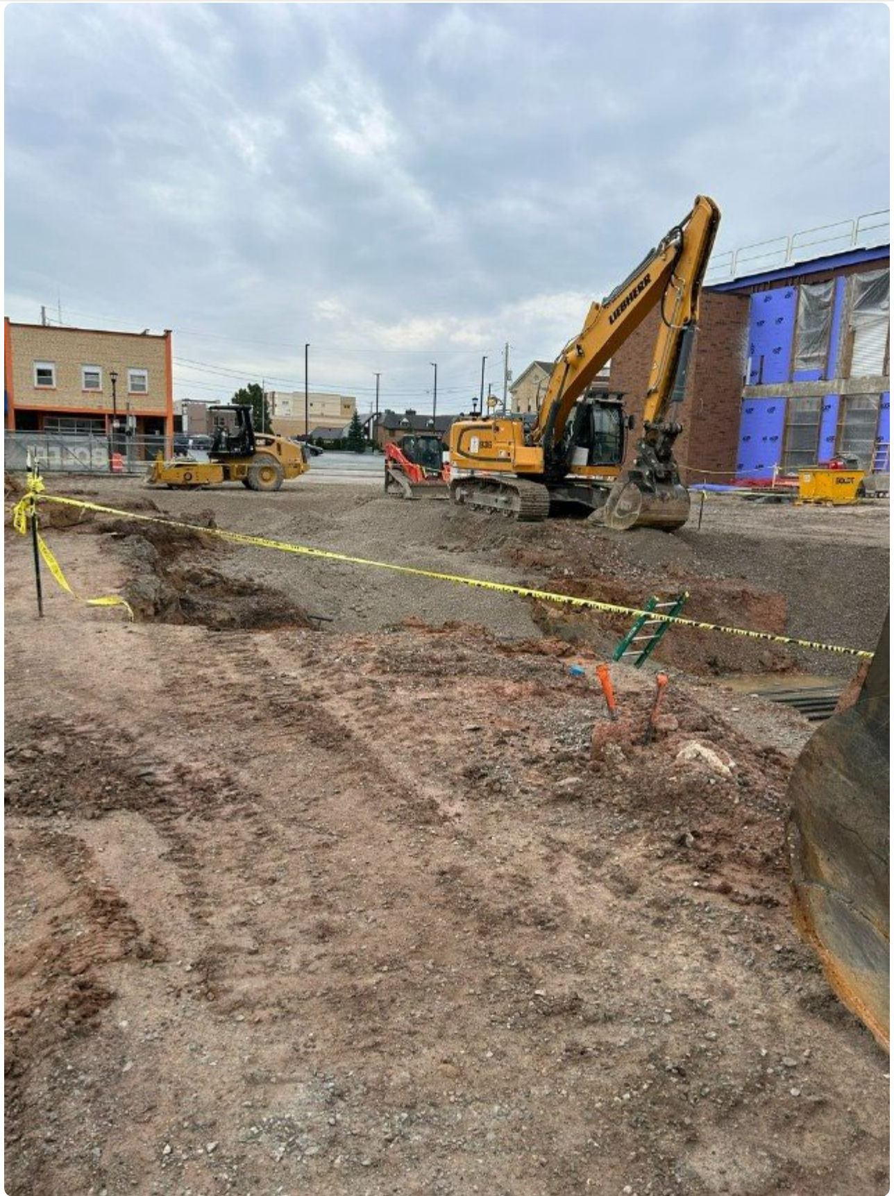
Geothermal Header Work
