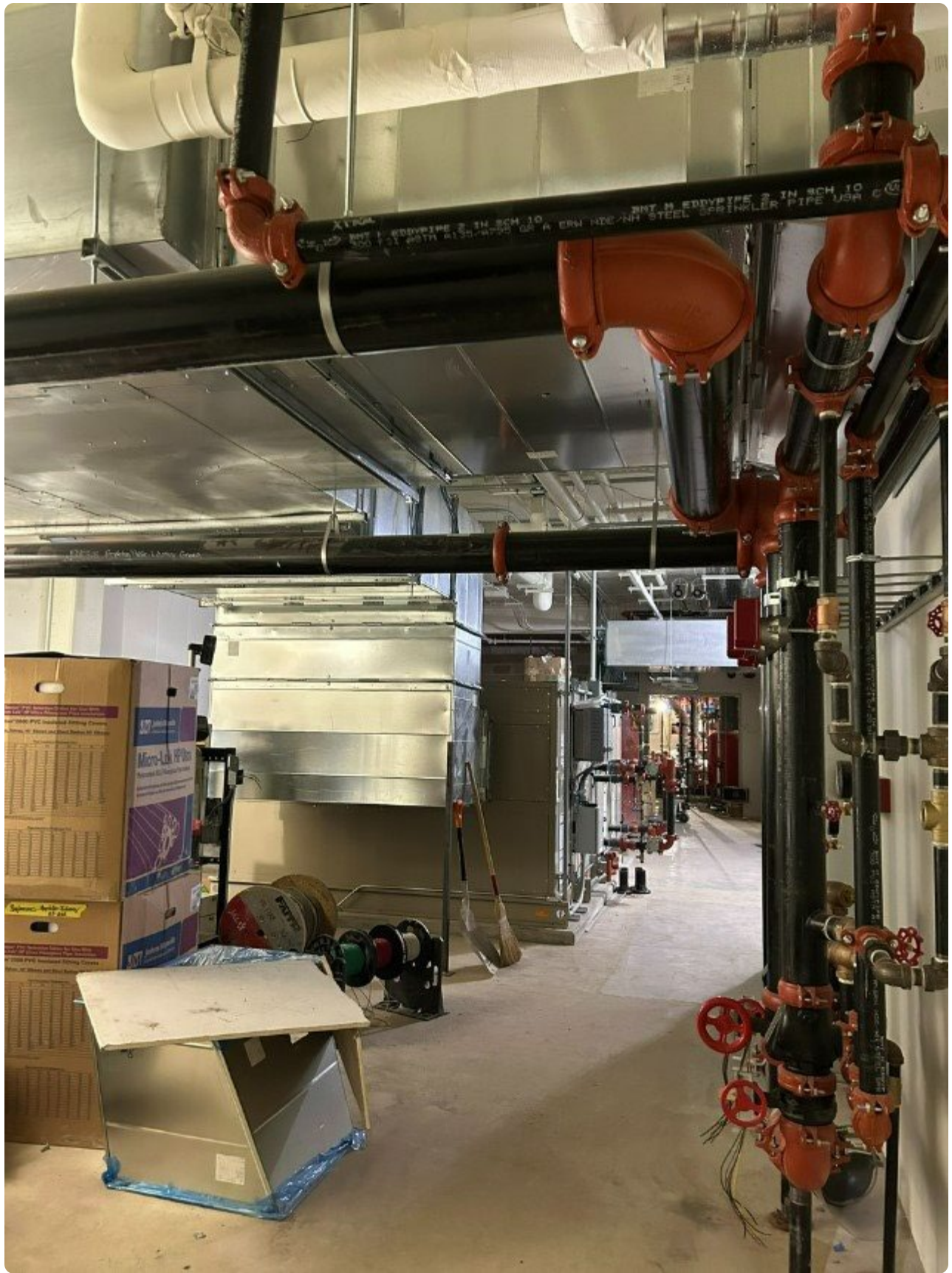
Lower-Level Air Handling Unit in Mechanical Room
