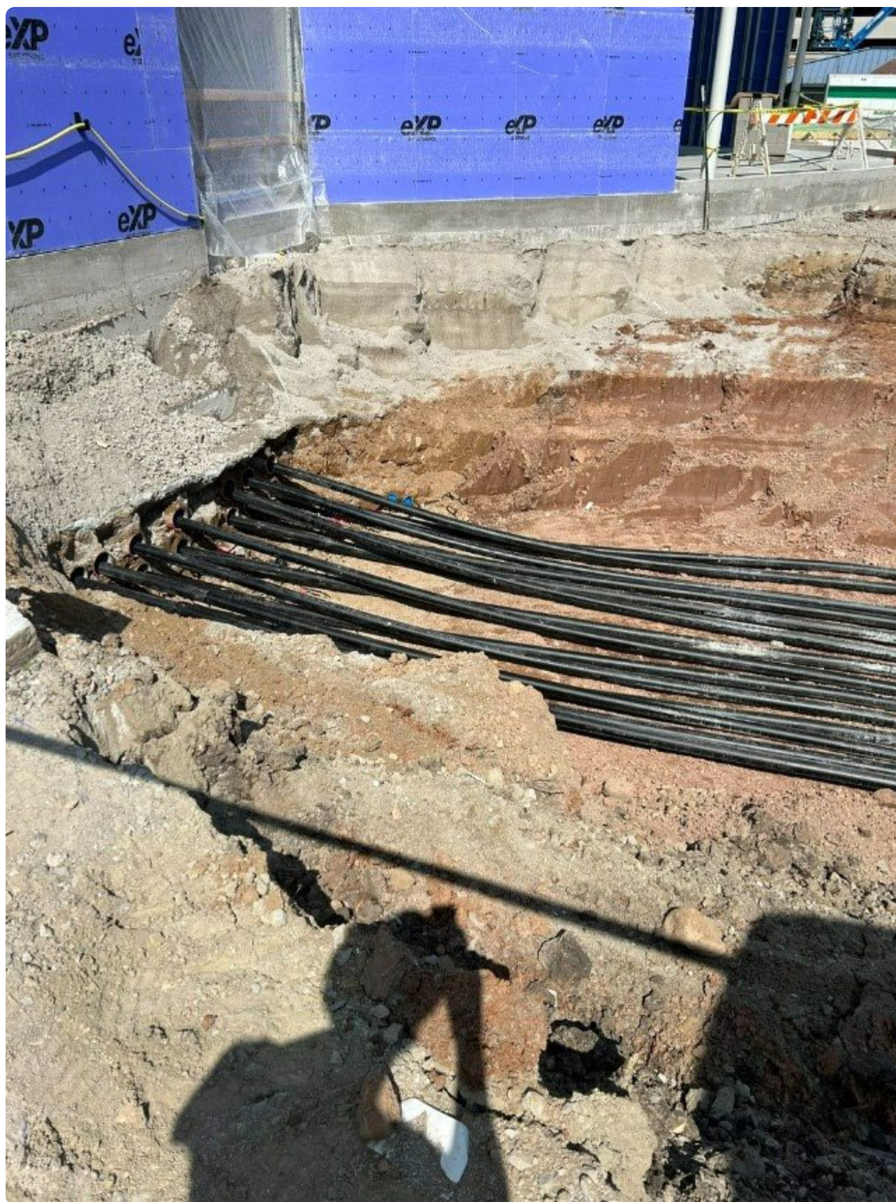
Geothermal Tubing from the Building to the Parking Lot
