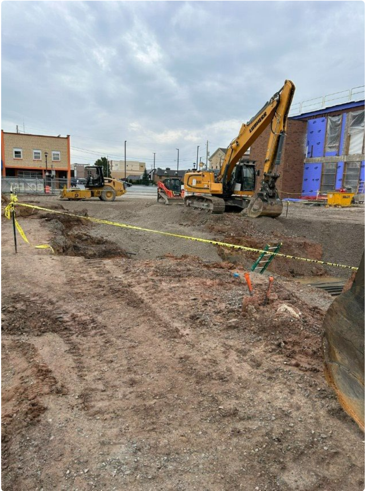
Geothermal Header Work
