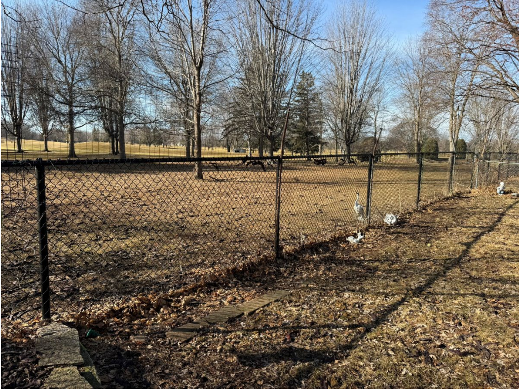
Our back fence is a 5' tall chain-link fence that we have extended with posts and wire fencing.
