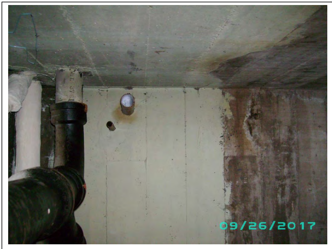
Photo 8 – View of probable fuel oil product and vent lines in west wall of boiler room.
