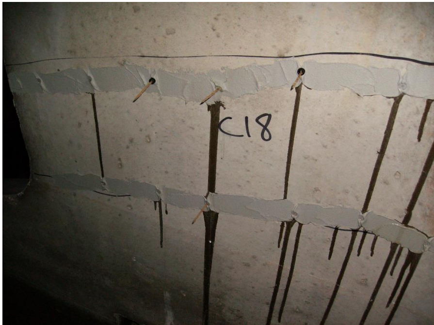
Photo 2 – Existing Epoxy Repair
