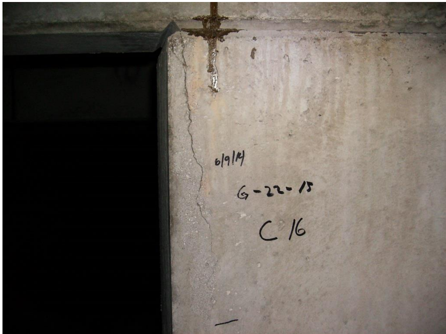
Photo 6 – C16, Side of crack shown not previously repaired.
