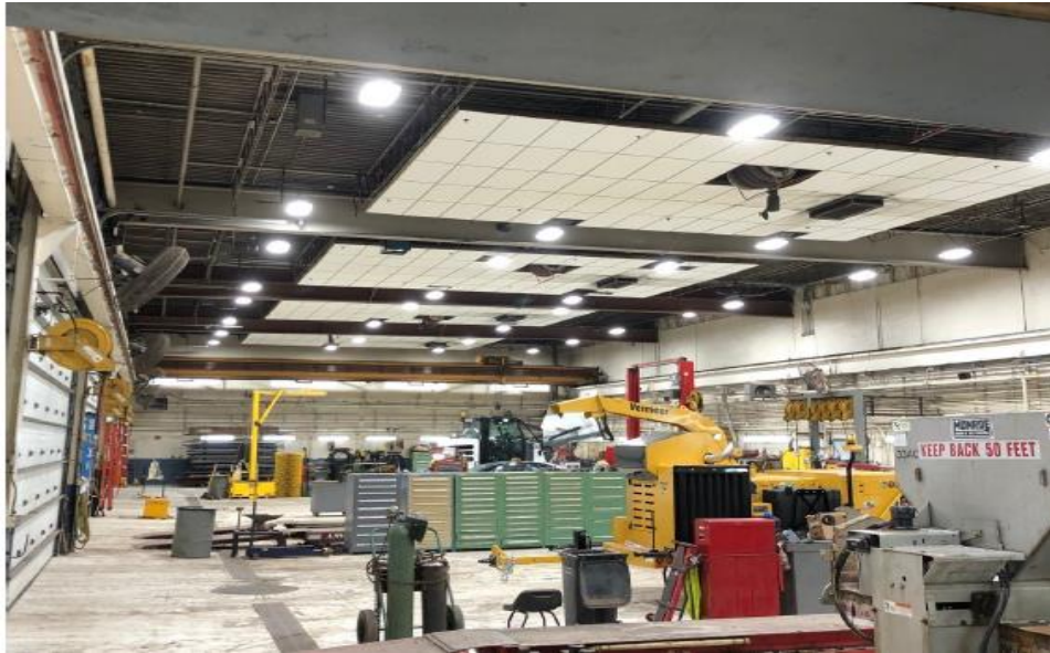
MSB CEA Mechanic Shop new LED fixtures installed
