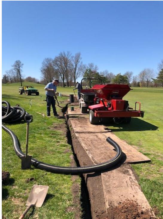
Utilizing the new topdresser/material hauler to back trench with pea gravel on #14.
