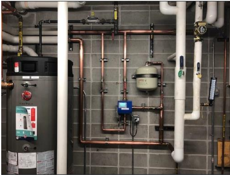
Police Station water heater, mixing valve, and piping replacement
