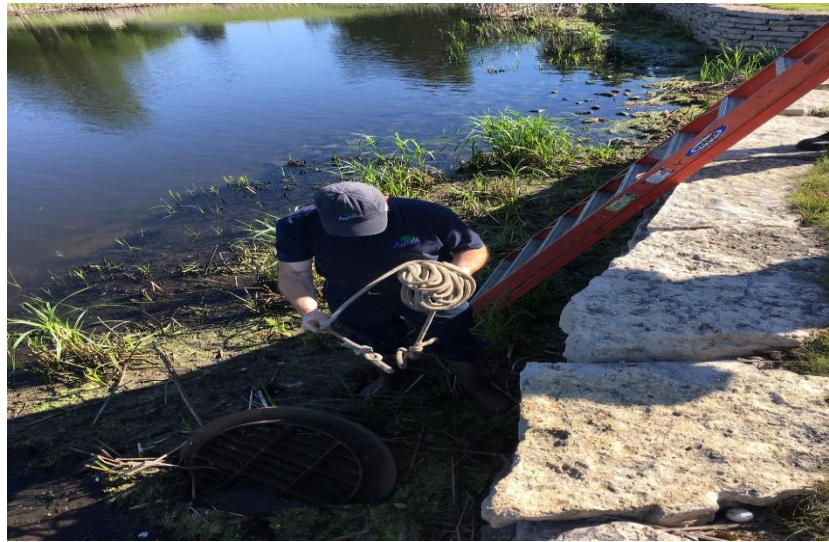
Jim Pedersen hooking up rope to pull catch basin lid from pond.
