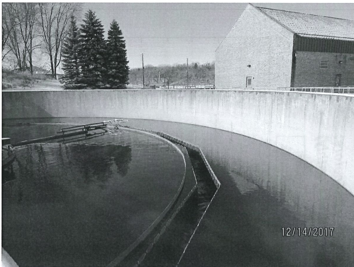
Close-up view of secondary clarifier
