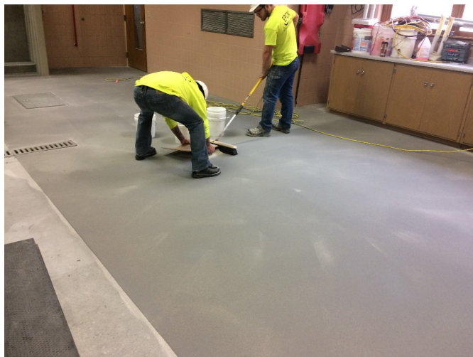
Contractor's working on the epoxy floor coating at Fire Station #4. Project has since been completed.
