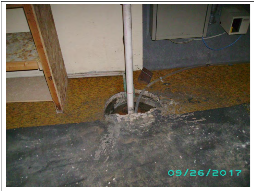
Photo 10 – View of sump drain along north wall of newer section of building.
