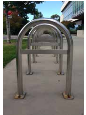
Staple racks provide secure parking options for bicycles, accommodating 2 points of contact and a U-Lock. See Appendix 6 for more detail on parking selection.
