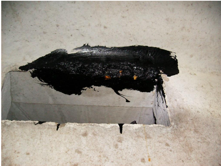
Photo 5 – E31, Minor corrosion at rebar coating.
