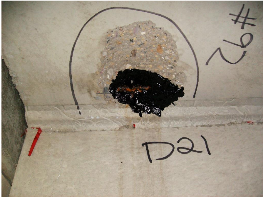
Photo 11 – D21, Minor corrosion at repair.
