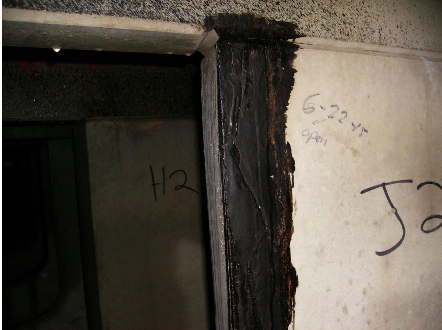
Photo 3 – J2, Open Crack at Repair
