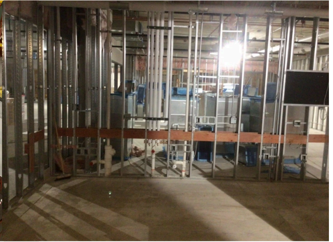
Room Framing on Lower Level
