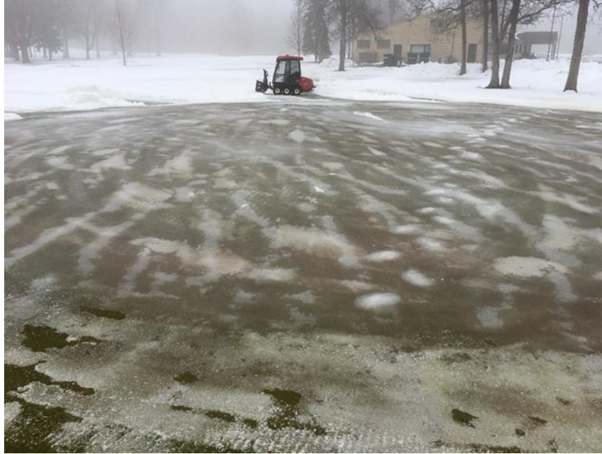
After snow removal on 1/19.
