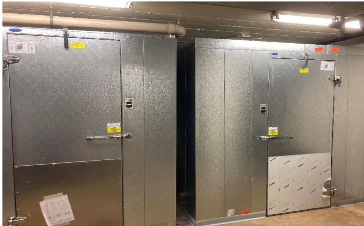
Freezer on left and cooler on right after installation.
