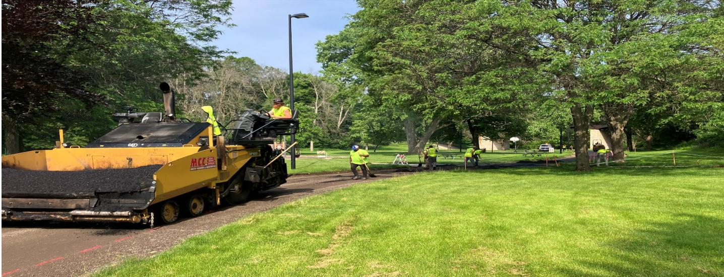
MCC removed the existing failing asphalt, brought in additional base, and paved the Highview Trail from Brookshire to Mead St.
