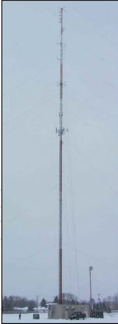
EXISTING TOWER PROFILE (LOOKING NORTHWEST)
