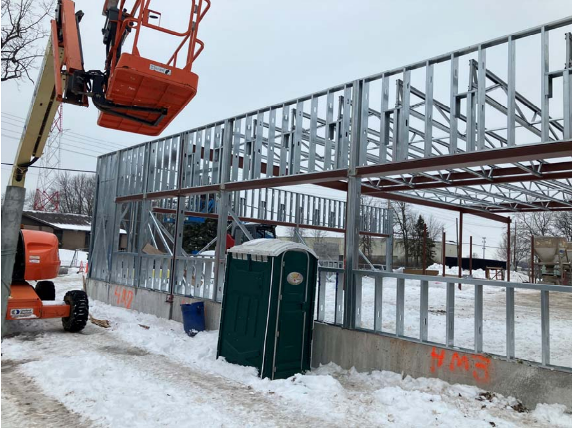
Figure 2: Valley Transit Whitman Ave facility renovation progress.
