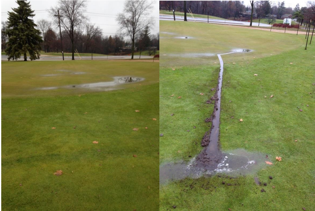
Above: before and after measures taken to remove surface water from #16 Green, preventing Winter ice damage. This is done after the course closes for winter and is repaired prior to course opening in Spring. This is done on two other greens where water can pocket too.
