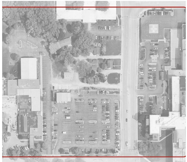
St. Elizabeth Hospital Parking Lot existing
