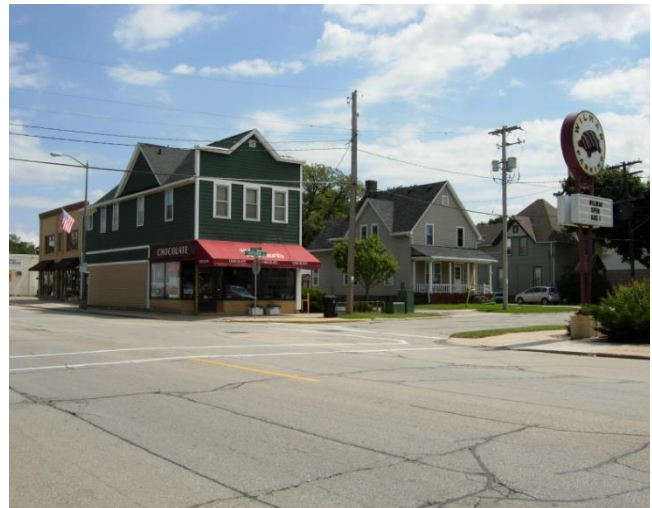
A remodeled building on Wisconsin Avenue
