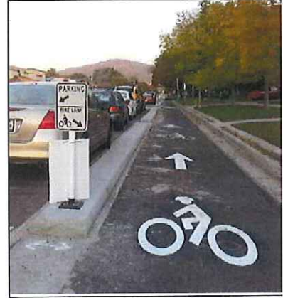
Figure 29: Bike Lane – Separated Separated bike lanes, sometimes called "cycle tracks" or "protected bike lanes," separate the bike lane from travel lanes with a vertical element such as curbs, bollards, pavement elevation, parked cars, or planters. While separated bike lanes increase bicyclists' sense of comfort, they still have conflict points at intersections and driveways, where turning traffic crosses them. Separated bike lanes may be placed at street level, sidewalk level, or an intermediate level, and may include vertical or rolled curbs.
