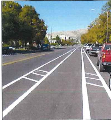
Figure 28: Bike Lane – Buffered Buffered bike lanes are standard bike lanes that include a painted buffer on one or both sides of the bike lane. This buffer provides increased separation between a bike lane and a motor vehicle travel lane or a parking lane. A typical bike lane and buffer combination is a 5 foot bike lane and a 2-3 foot buffer. A buffer next to travel lane ensures that motorists give bicyclists the minimum 3-foot clearance when passing. A buffer next to parked cars helps to keep bicyclists from riding in an area where car doors may open into their paths.
