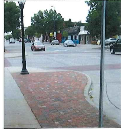
Figure 22: Pedestrian Bump-out / Curb Extension Curb extensions reduce the effective street crossing distance for pedestrians by narrowing the streets. They also have a minor impact on reducing traffic speeds by narrowing the street. Curb extensions can also provide space for bicycle racks, benches, or other amenities.
