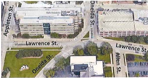
Figure 4: Oneida Street and Lawrence Street Intersection The Oneida Street and Lawrence Street intersection is one of the most confusing in downtown Appleton.
