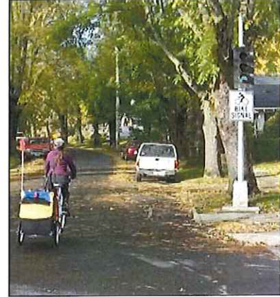
Figure 38: Bike Signal Bicycle signals are traffic signals that govern bicycle movements at an intersection. Bicycle signals may be used when bicycles, pedestrians, and motor vehicles have different movement cycles.
