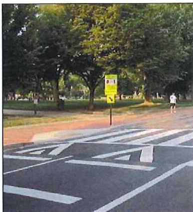
Figure 23: Raised Crosswalk Raised crosswalks are elevated from the street level, typically to the level of the curb and sidewalk. Raised crosswalks are essentially speed tables with a flat top that is wide enough for a crosswalk. Raised crosswalks encourage motorists to yield to pedestrians because the raised crosswalk increases pedestrian visibility and forces motorists to slow down before going over the speed table. Raised crosswalks may eliminate the need for pedestrian ramps at intersections. Street drainage must be carefully considered when retrofitting raised crosswalks.
