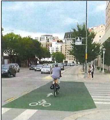
Figure 36: Colored Pavement Green colored pavement may be used to increase the visibility of bicycle facilities. Colored pavement may be used to highlight an entire bicycle corridor, but is most useful to highlight bicycle facilities in conflict areas – through intersections, across driveways, or crossing highway ramps.
