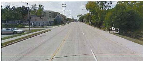
Figure 48: Packard Street – Existing Conditions
