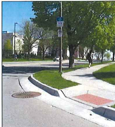
Figure 18: Crosswalk: Unmarked In Wisconsin, unmarked crosswalks are the continuation of a sidewalk on one side of the street to the other side of the street. Motorist must always yield the right of way to pedestrians in any unmarked or marked crosswalk except at a signalized intersection where pedestrians follow the appropriate signal.
