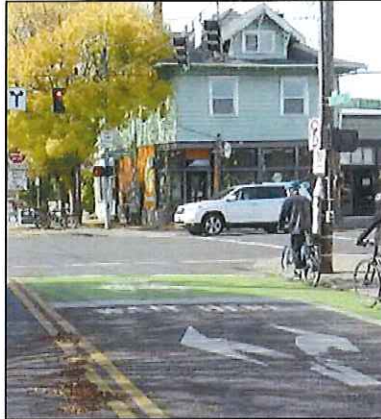
Figure 37: Bike Box A bike box is a designated area at the front of a traffic lane at a signalized intersection. Bike boxes provide bicyclists with a location to wait for a green signal that puts them in a location visible to motor vehicle traffic also stopped at the intersection. Bike boxes can facilitate left turns for bicyclists and can reduce the likelihood of “right-hook” crashes with turning vehicles. Bike boxes can also benefit pedestrians as they reduce vehicle encroachment in crosswalks. Installation of bike boxes also requires installation of “No Turn on Red” signs.
