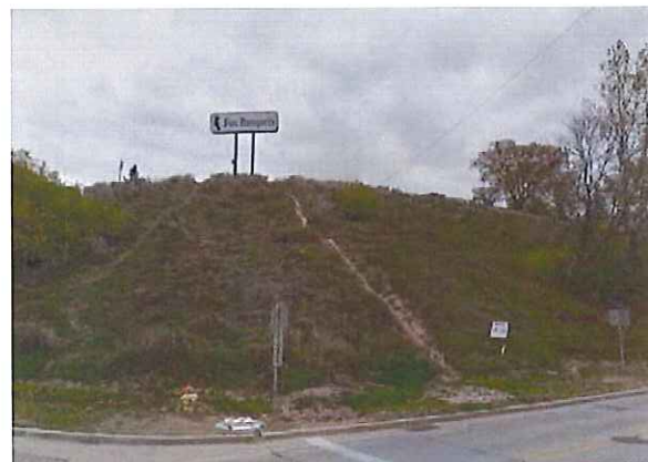
Figure 45: Existing Conditions – Location of Proposed Staircase
