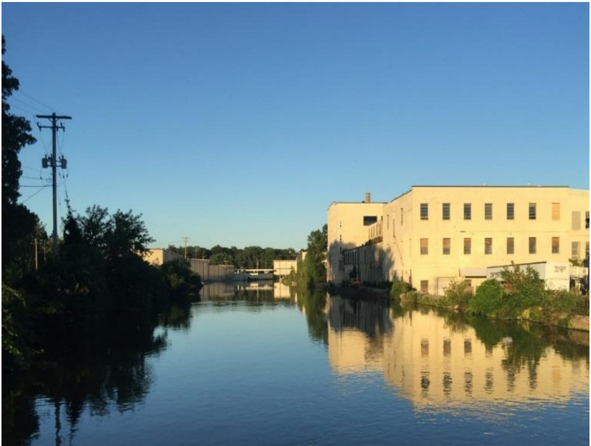
Figure 1 A significant share of new housing development has occurred along the Fox River. The Woolen Mills project is converting a century-old mill into 60 apartment units, contributing to the growth of a vibrant mixed-use neighborhood once dominated by heavily industrialized uses.
