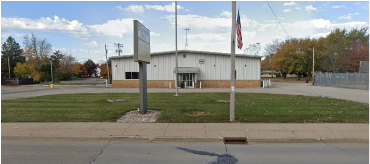
Richmond Hall existing condition
