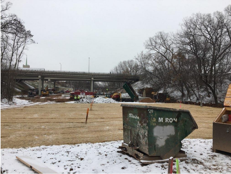
Looking south towards performance stage that is currently under construction.
