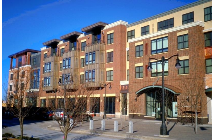
Figure 13 Stacked flats, St. Louis Park, Minnesota
