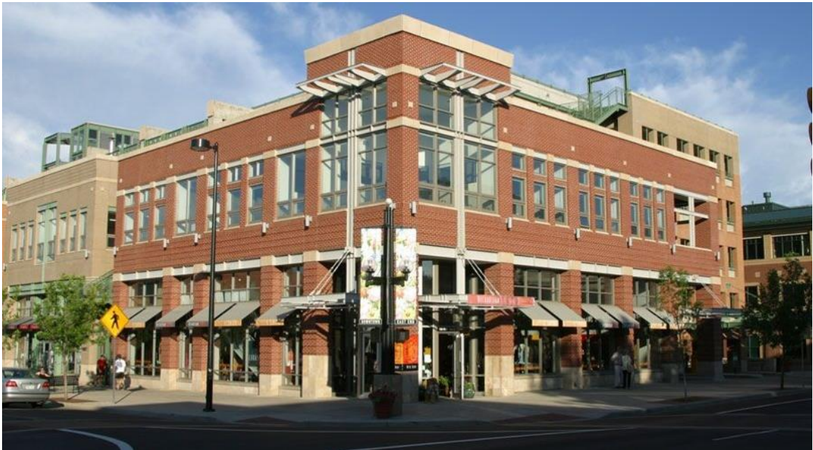
Figure 52 Mixed use parking structure with liner shops. While mixed use parking structures have been successfully developed in some cities, insufficient market demand has undermined their economic viability in others.
