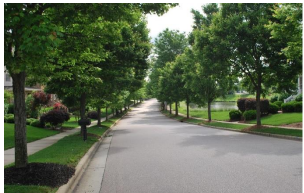
Figure 26 Example of well-designed and maintained residential streetscape
