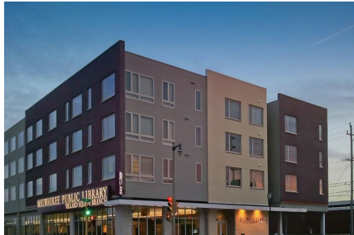
Figure 64 New libraries are often built as mixed use projects, such as the Willard Square Branch library in Milwaukee, which incorporates housing
