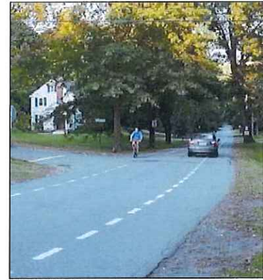
Figure 32: Bike Lane – Advisory Many lower-traffic roads are too narrow to provide exclusive space for two standard-width bicycle lanes and two standard-width travel lanes. For lower volume, lower speed roads, advisory bike lanes (ABLs) have been developed as an alternative to a shared lane marking treatment to separate bicyclists from automobile traffic. These roads are marked to provide two separate standard width bicycle lanes on either side of a single shared (un-laned) motor vehicle travel space essentially creating a three-lane cross section. Roadway centerlines are not present. Parking lanes may be provided outside the advisory bike lanes.
