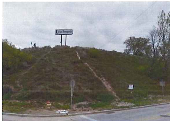
Figure 45: Existing Conditions – Location of Proposed Staircase
