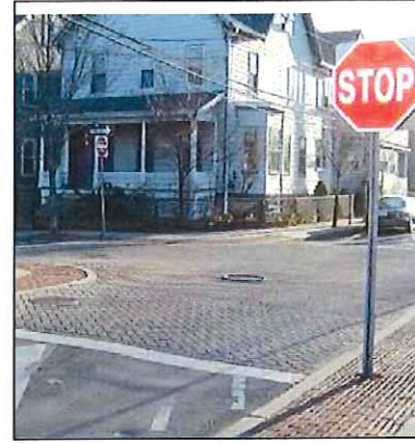
Figure 16: Raised Intersection Raised intersections elevate an entire intersection to the level of the curb and sidewalk, essentially creating a large speed table. Like raised crosswalks, raised intersections encourage motorists to yield to pedestrians because the raised intersection increases pedestrian visibility and forces motorists to slow down before going over the speed table. The crosswalks on each approach to a raised intersection are also elevated to enable pedestrians to cross the road at the same level as the sidewalk, eliminating the need for curb ramps. Raised intersections may use standard paving materials such as concrete or asphalt, or may use materials such as brick or other pavers to further differentiate the space.
