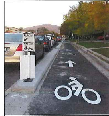
Figure 29: Bike Lane – Separated Separated bike lanes, sometimes called "cycle tracks" or "protected bike lanes," separate the bike lane from travel lanes with a vertical element such as curbs, bollards, pavement elevation, parked cars, or planters. While separated bike lanes increase bicyclists' sense of comfort, they still have conflict points at intersections and driveways, where turning traffic crosses them. Separated bike lanes may be placed at street level, sidewalk level, or an intermediate level, and may include vertical or rolled curbs. Preferred Width: 6.5 feet plus gutter pan (one way); 10+ feet plus gutter pan (two-way) Minimum Width: 5 feet plus gutter pan (one-way); 8 feet plus gutter pan (two-way)
