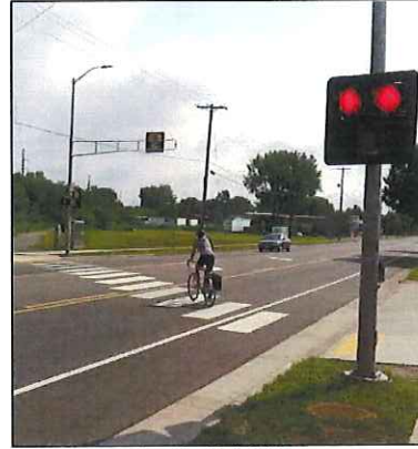
Figure 19: Pedestrian Hybrid Beacon ("HAWK") A pedestrian hybrid beacon is an overhead warning device, used at locations that are unusually hazardous or where pedestrians or bicyclists should be expected to cross throughout the day or where pedestrian crossing activity would not be readily apparent. The beacon is dark until activated by a pedestrian or bicyclist. When activated, the beacon displays a yellow signal followed by a red signal to drivers and a "walk" signal to pedestrians. Criteria for installation are available in the MUTCD.
