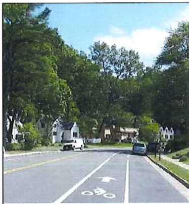
Figure 27: Bike Lane – Standard Standard bike lanes are signed and marked with pavement markings to designate space for bicyclists outside of the travel lanes to minimize conflicts on busier streets. Bike lanes typically operate in the same direction as motor vehicle traffic. Bike lanes are best suited for two-way arterial and collector streets where there is enough width to accommodate a bike lane in both directions. On one-way streets, they may be located on either the right or the left side of the roadway. Preferred Width: 5 feet plus gutter pan; 6 feet with integral curb and gutter; 6+ feet next to parking Minimum Width: 4 feet plus gutter pan; 5 feet with integral curb and gutter; 5+ feet next to parking
