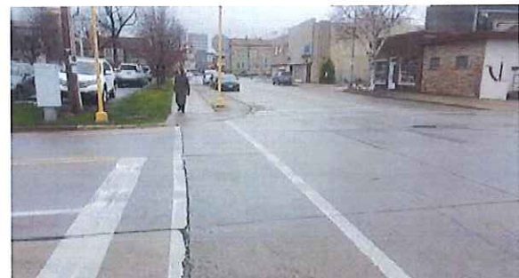
Figure 10: Downtown Area Crosswalk Crosswalks in the downtown area lack visibility.
