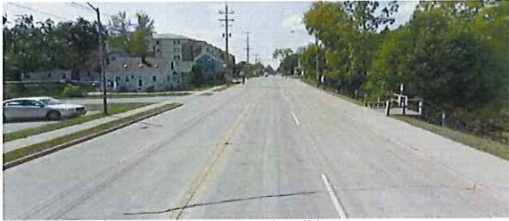
Figure 48: Packard Street – Existing Conditions
