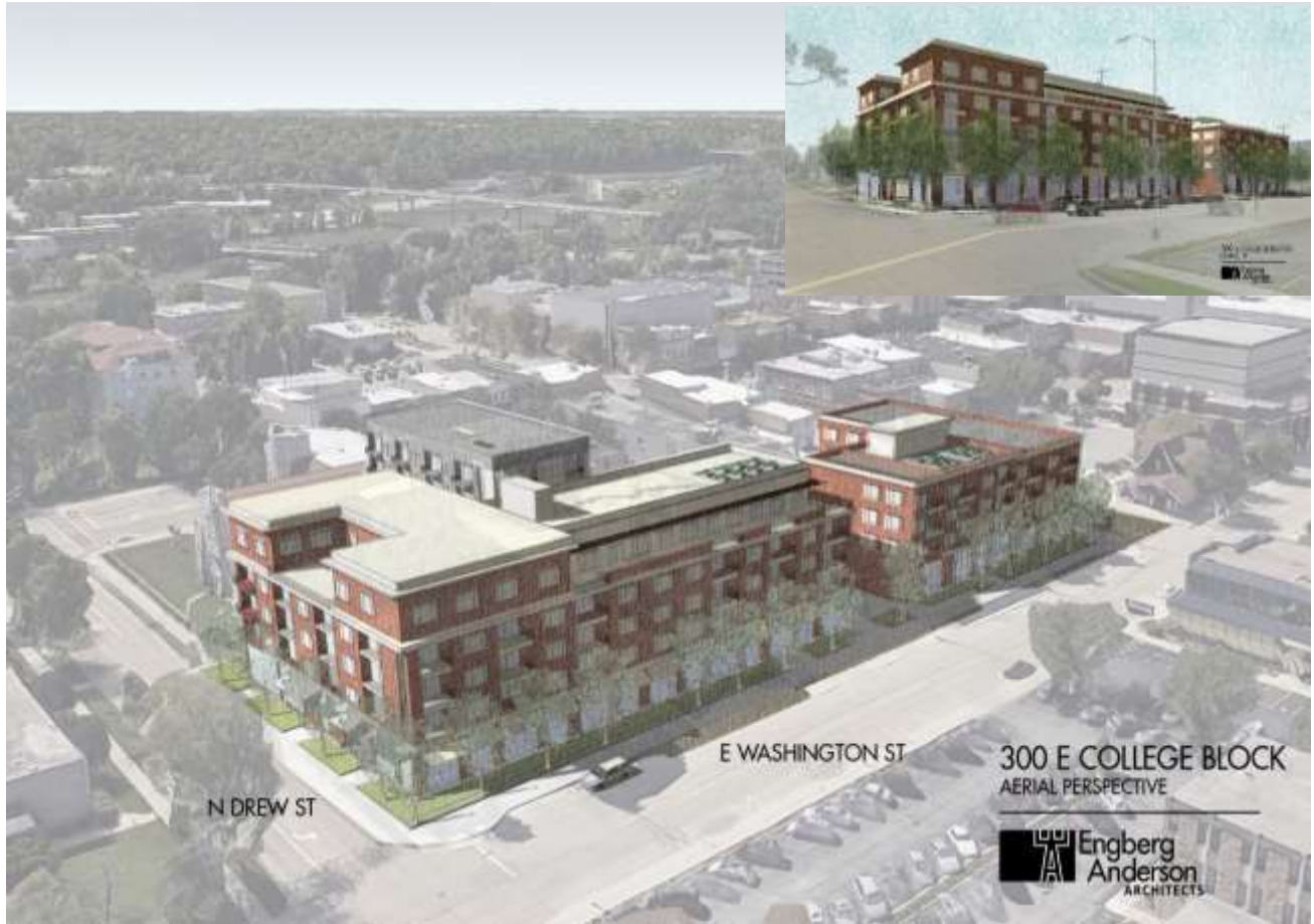
PERSPECTIVE OF CONCEPTUAL REDEVELOPMENT OF 300 BLOCK OF E. COLLEGE AVENUE VANTAGE POINT IS LOOKING SOUTHWEST TOWARD THE FOX RIVER FROM THE CORNER OF N. DREW STREET AND E. WASHINGTON STREET.
