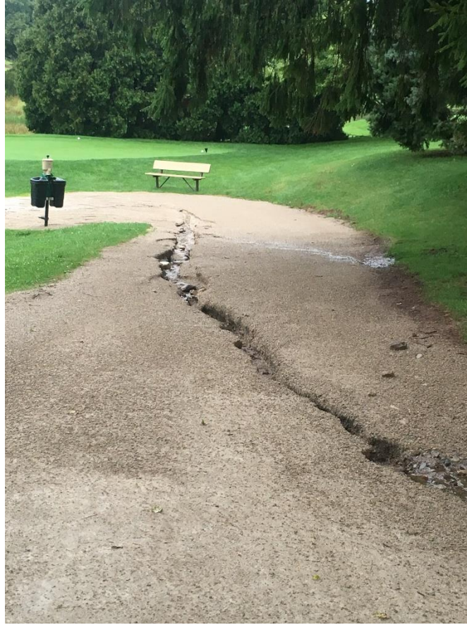
Cart path from #12 green leading to #13 tee washed out after a heavy rain.
