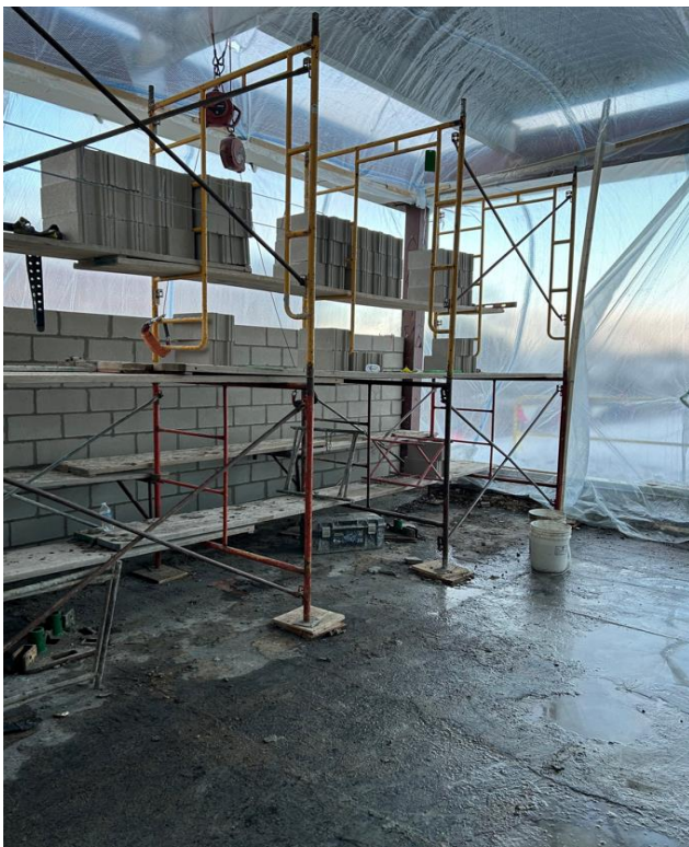
Freight Elevator – Upper Level
