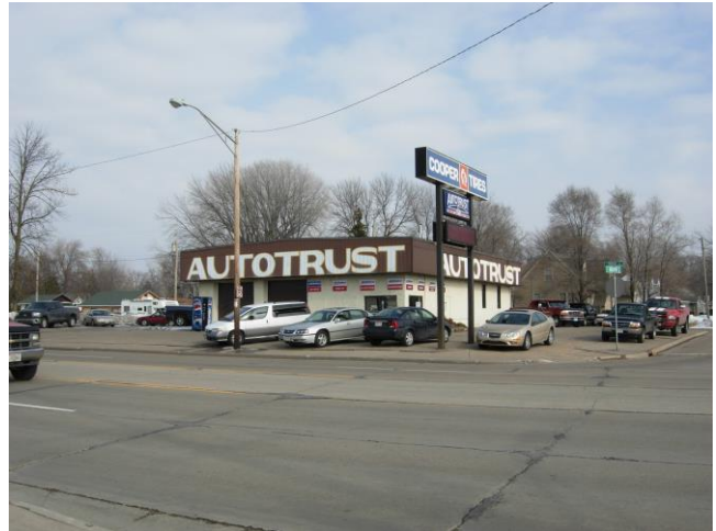
Example of a building that does not meet the City's standards for new construction.
