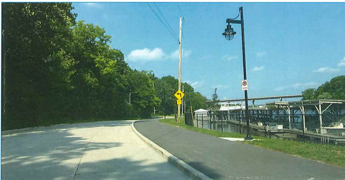
Figure 1 - Lutz Park Multi-Use Trail (as constructed)
