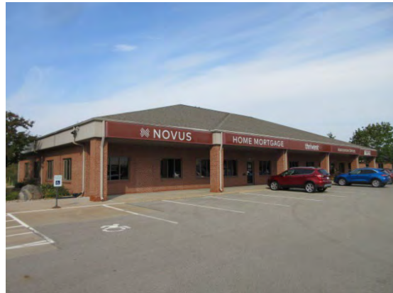
Typical Exterior View
