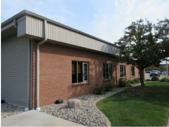
Typical Exterior View
