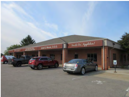
Typical Exterior View
