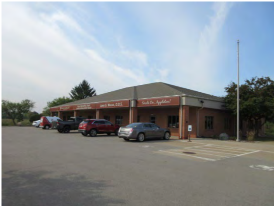
Typical Exterior View
