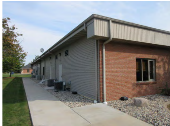
Typical Exterior View
