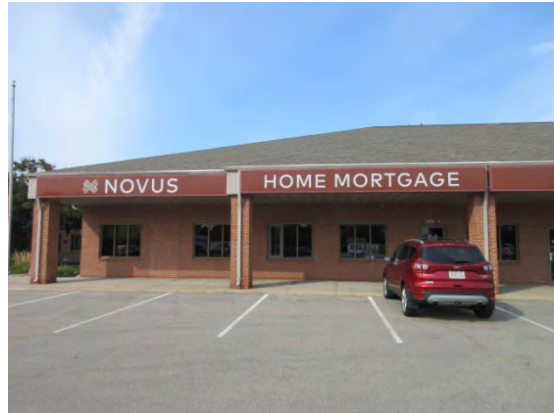
Typical Exterior View
