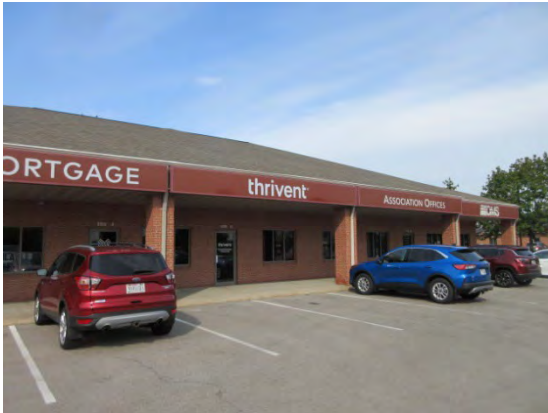
Typical Exterior View
