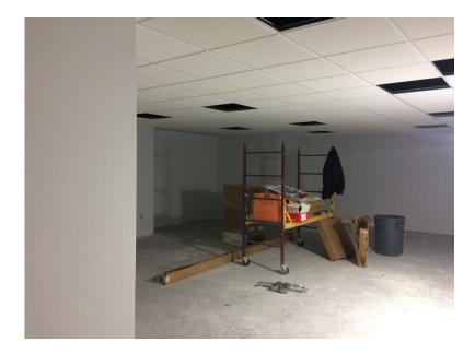
Renovation of a room previously known as the ozonator. The equipment was removed to reutilize the space. This space contained asbestos which was also fully remediated.
