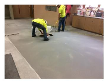
Contractor's working on the epoxy floor coating at Fire Station #4. Project has since been completed.
