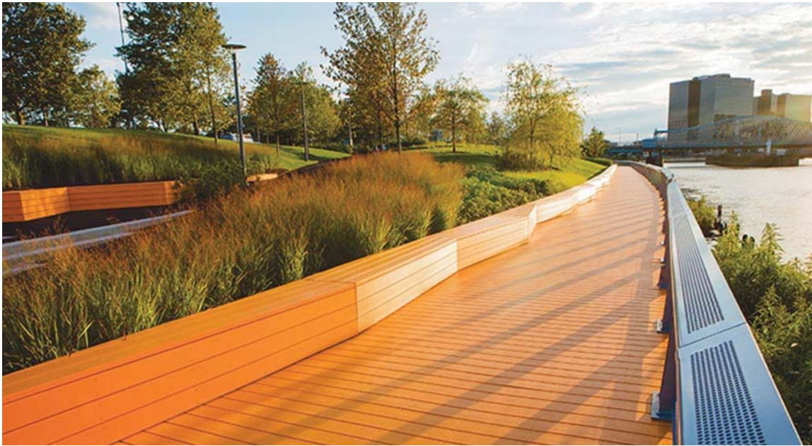
Cantilevered boardwalk as a designed landscape
