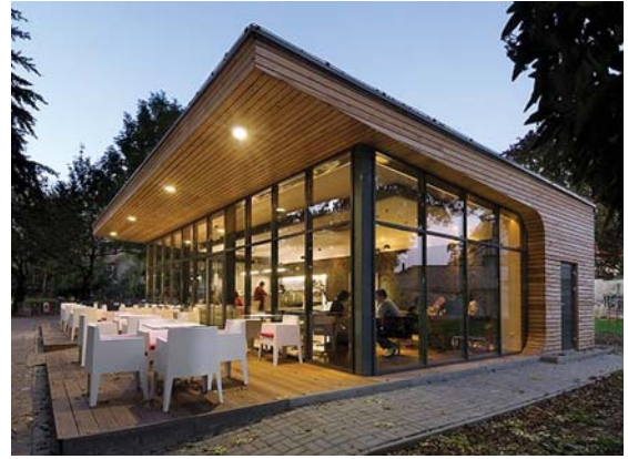
Room with glass walls
