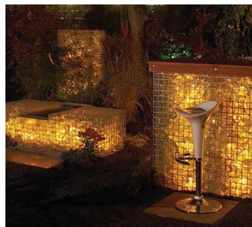
Tumbled Glass with interior lighting in gabion
