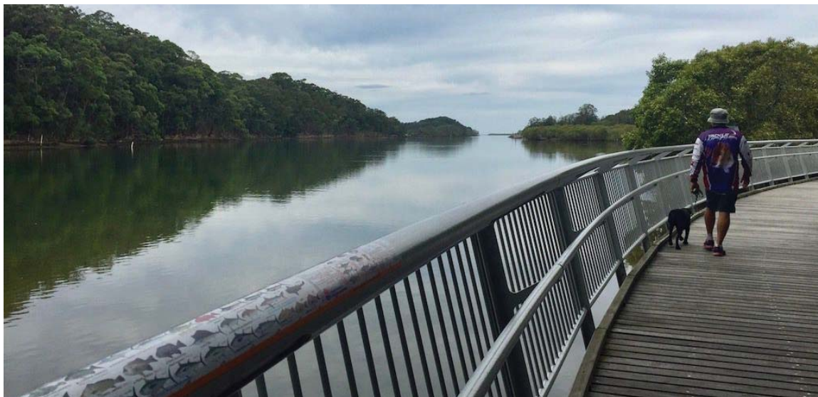
Pile supported boardwalk with interpretive fish sign
