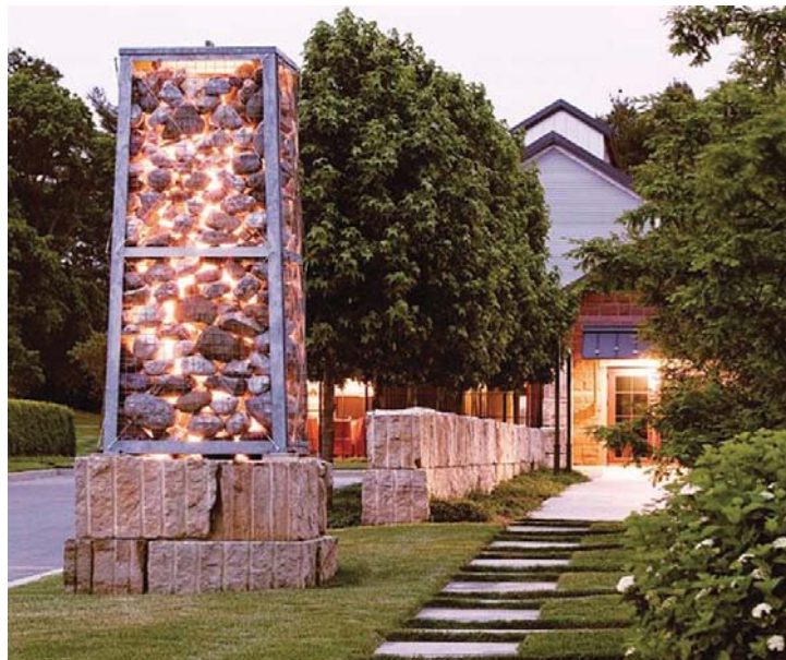
Stone gabion column internal lighting
