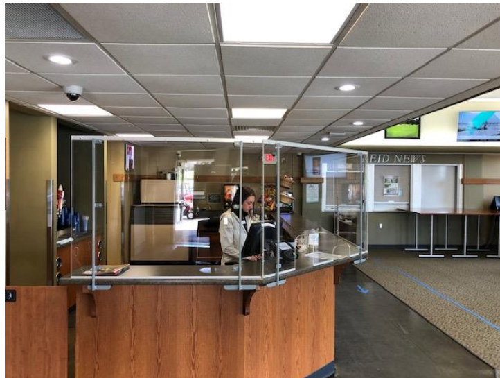
New Plexiglas installed at counter for staff and customer safety, similar sections were added in pro shop.
