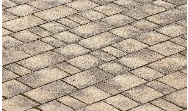
Permeable Paving
