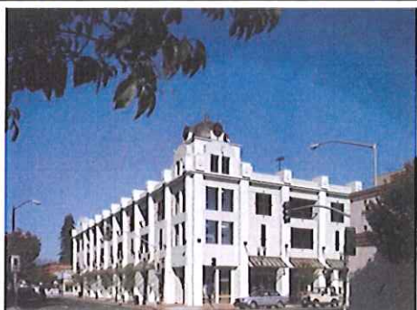
Mixed-Use Public Parking Ramp City of Watsonville, CA
