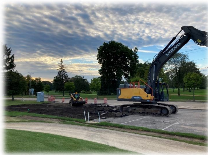
Work begins on parking lot near #17 tee.
