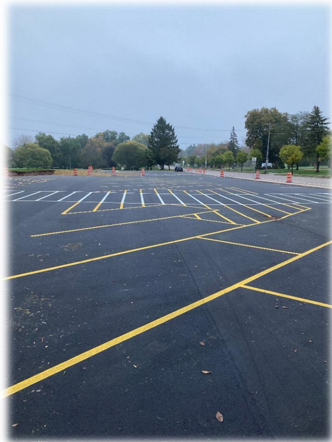
Finished parking lot looking east from west entrance.
