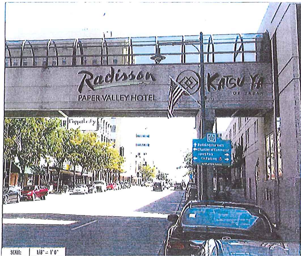
WEST LOCATION VIEW
