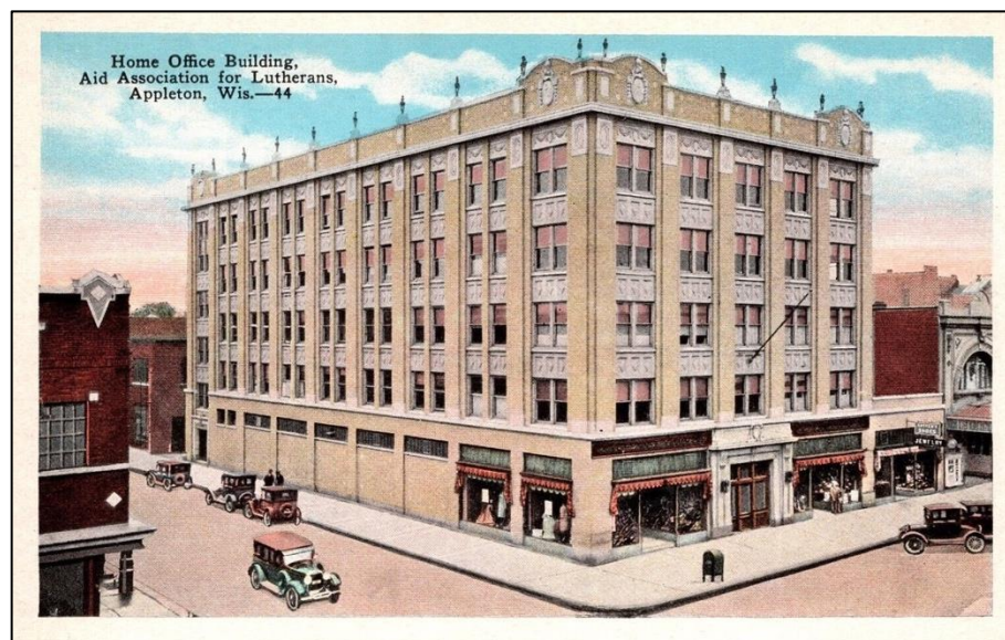
Figure 15. 1920s view of the Insurance Building, AAL's 1923 home office on the site of the current AAL Building and demolished in 1963. Source: Ebay.
