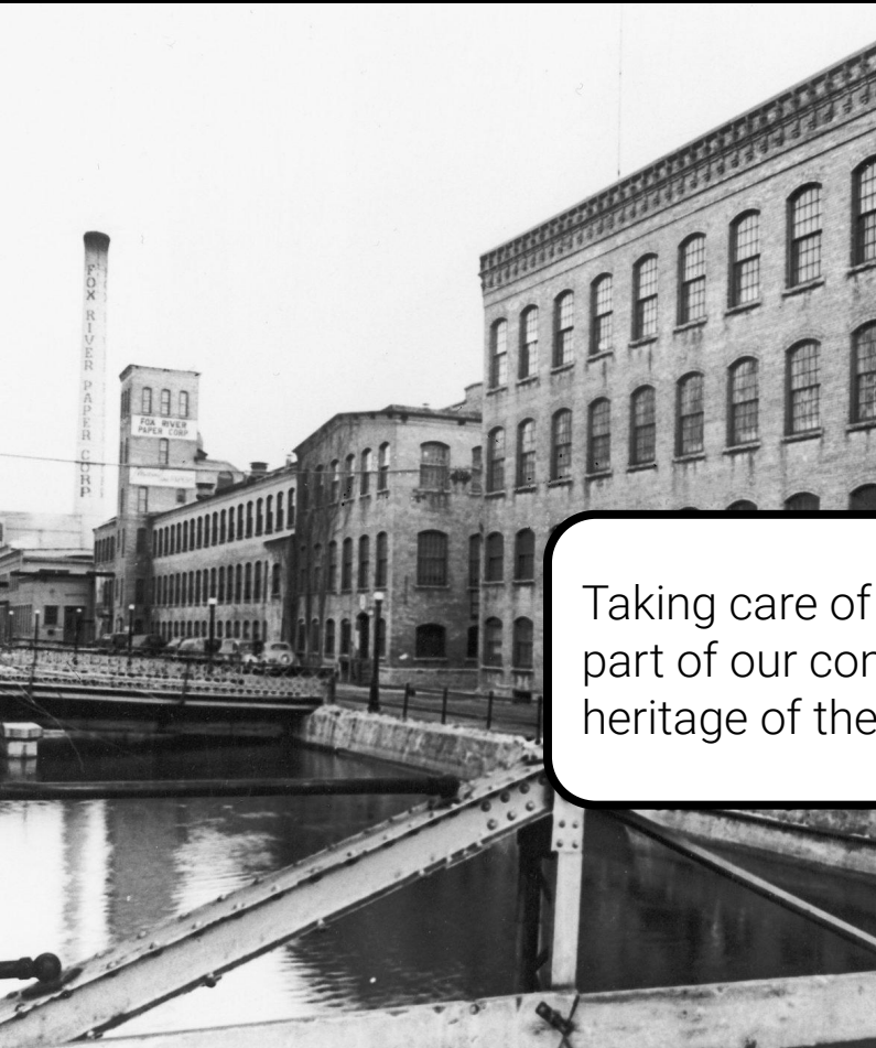
Fox River Mills, built in 1883 to 1915 Recently converted to Residential
