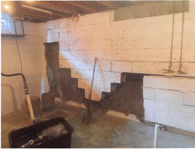
Car door sized holes in our foundation
