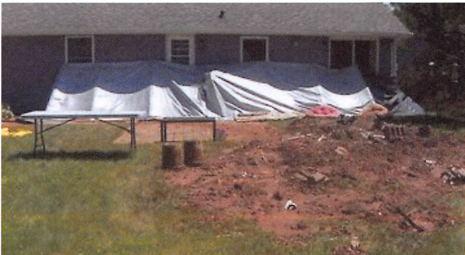
Tarps to protect exposed foundation
