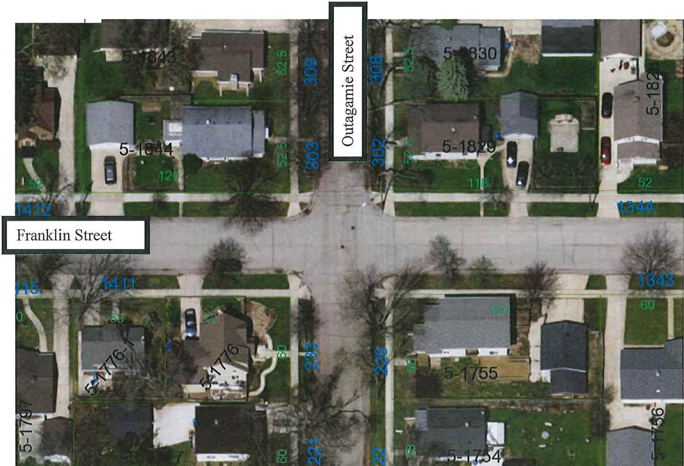
Aerial Photo, Intersection of Franklin Street & Outagamie Street
