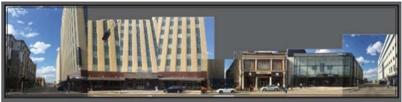
200 West College Avenue (north side) Chase Bank to 222 Building
