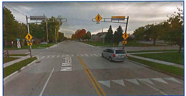
Push-Button Activated Strobe Light System (example) (to be installed at Evergreen/Meads) in 2019)
