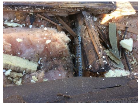
Replacement of roof at Fire Station #5
