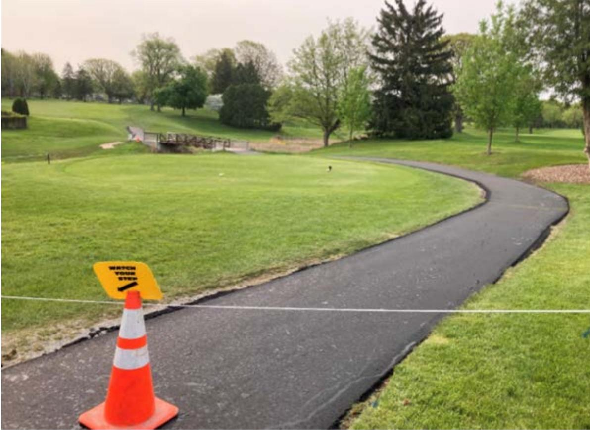
**Figure 11: Water Treatment Plant hardscape replacement.**
