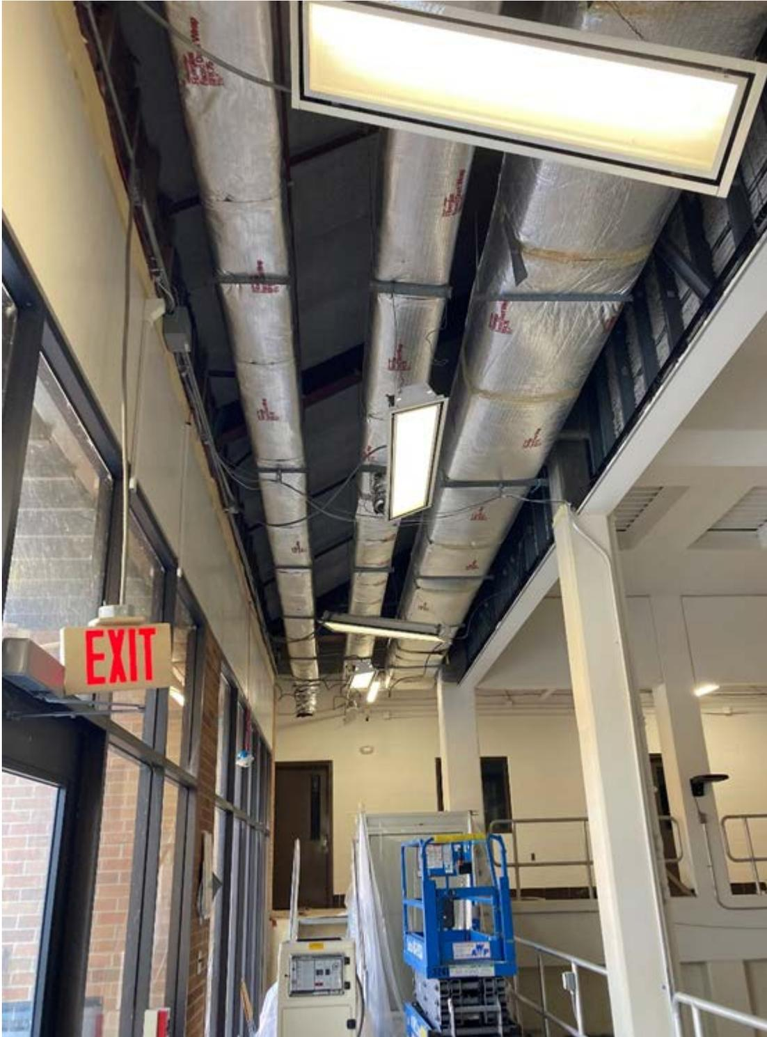
**Figure 14: Wastewater Treatment Plant HVAC upgrades for H & J buildings.**
