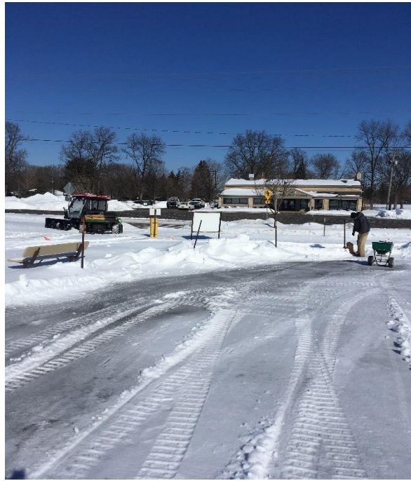
After removing snow black sand was added to absorb sunlight and melt the ice.
